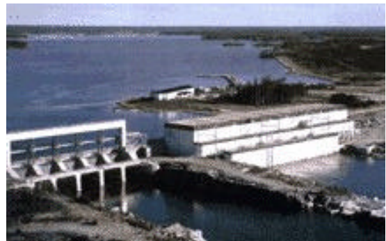
Jenpeg Generating Station
